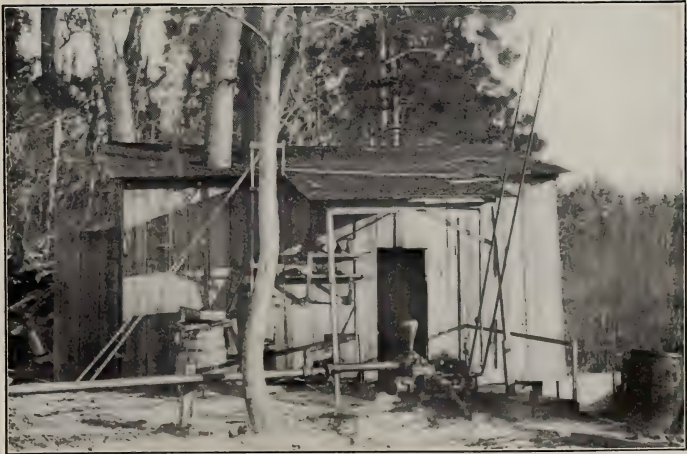
Fig. B. A temporary steam pumping plant on a lake-shore in Florida.
